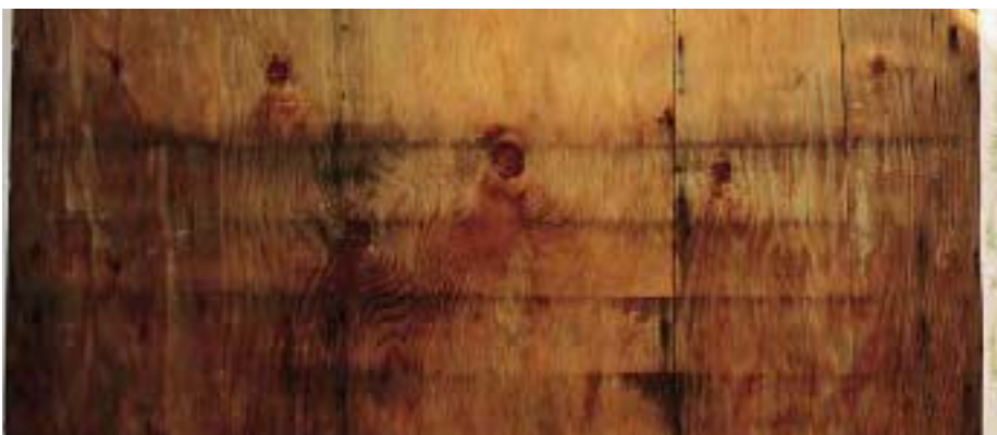
Figure 2. Highly permeable housewraps allow water vapor to escape to the exterior, helping walls to dry. However, in some circumstances, they can also allow water vapor to be driven inward, wetting the sheathing. Sun shining on damp wood siding can drive water vapor through a housewrap into the wall. These photos show water stains on the housewrap (top) and the sheathing (bottom) of a house with clapboard siding that had not been back-primed. The back side of the sheathing was dry, indicating that the moisture had traveled from the outside in. Although none of the sheathing on this house had rot, the siding paint peeled prematurely.
