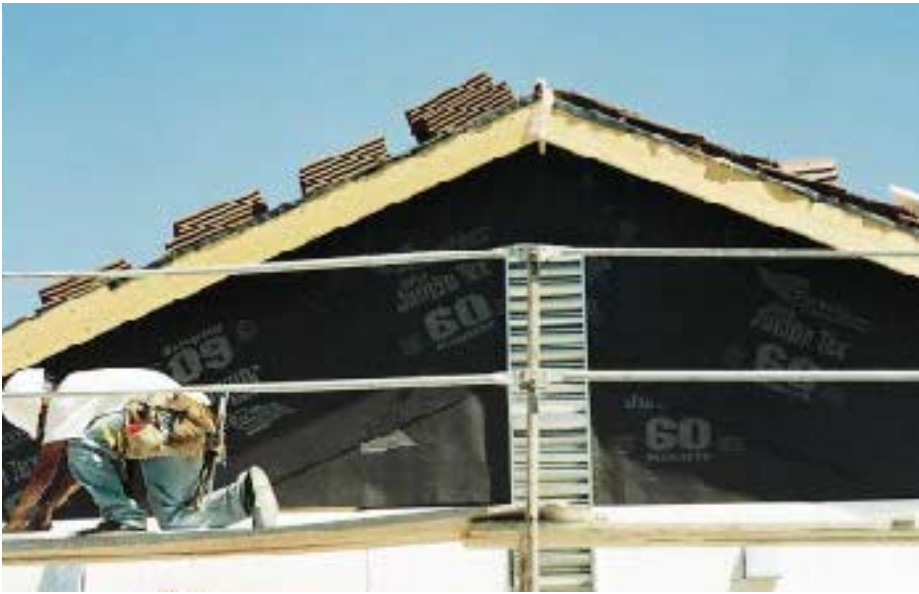
Figure 3. Grade D building paper is similar to asphalt felt, but lighter. It is made from virgin wood pulp, while asphalt felt is made from recycled cardboard.
